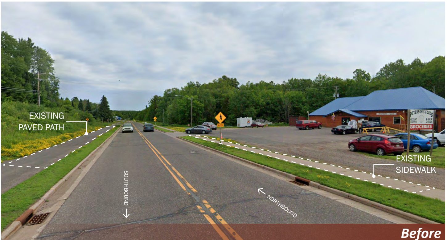
Figure 54 | Peterson's Crossing is a high-traffic stop along State Highway 13. A paved path runs alongside the southbound lane, while a concrete sidewalk serves northbound pedestrians. However, pedestrian signage is limited, and the area lacks pavement markings and curb cuts, creating accessibility and safety concerns. (Terra Soma)
