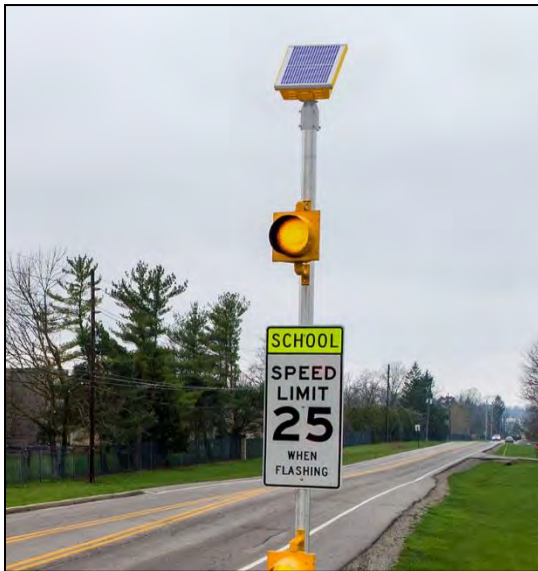
Example of proposed speed limit monitoring device using solar power for school zone. (USDOT)
